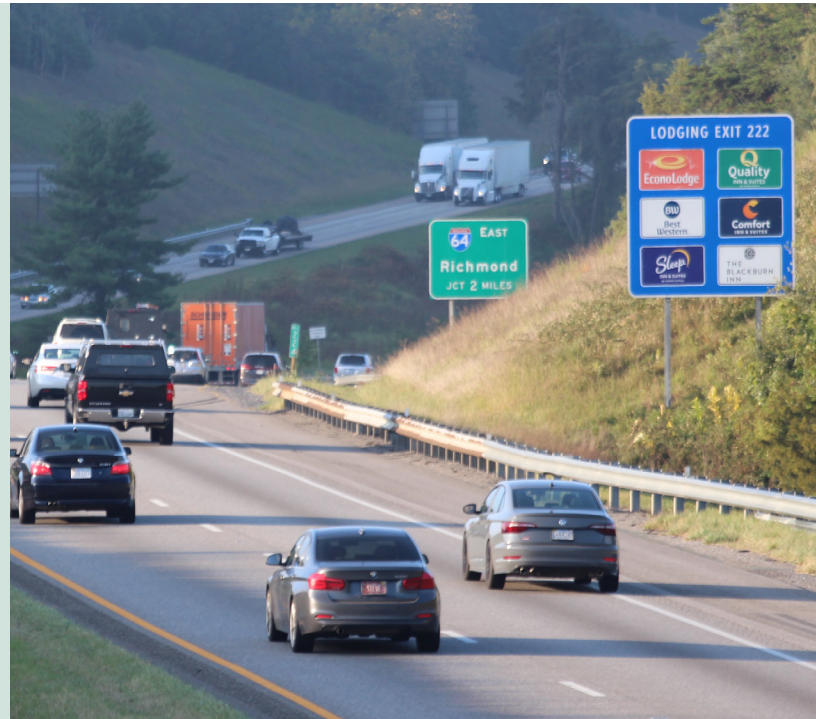
The widening of I-81 near Staunton is set to begin in spring 2024.
