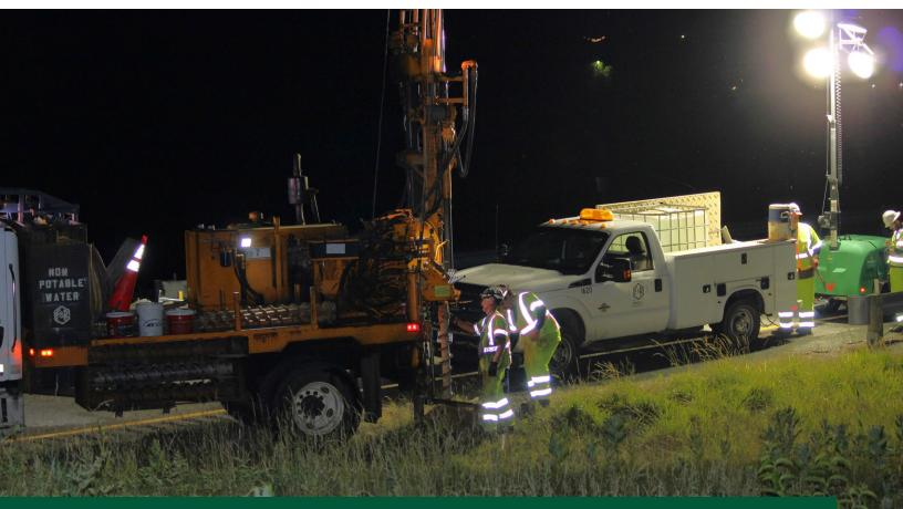
Nighttime work along I-81 in the Staunton area includes drilling for soil and rock samples
